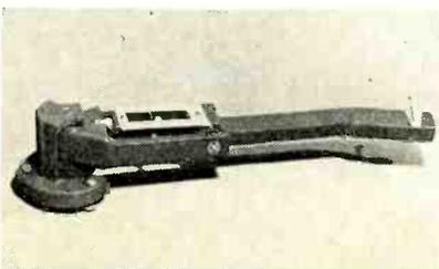
new arms are fabricated from magnesium and have a precision ground angular-contact ball pivot. Without cartridge the arms are priced at \$35.
