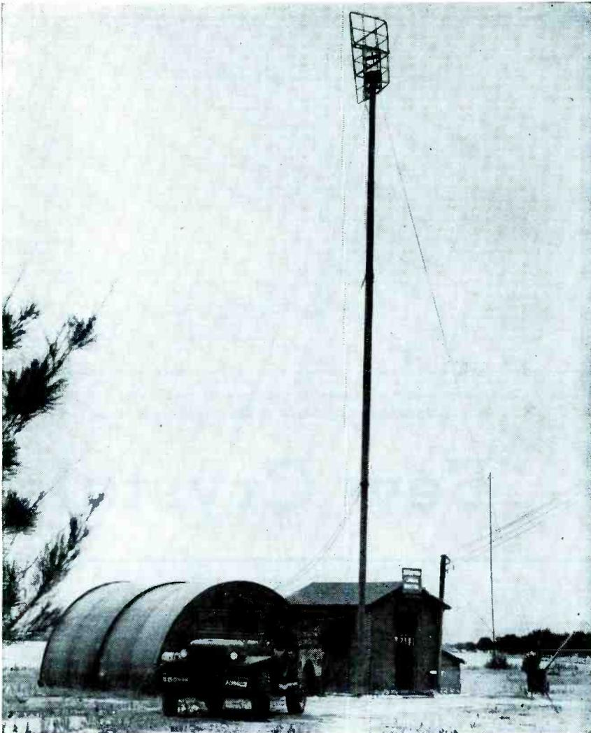
Typical shoran ground station as set up by surveying crew, using 50-foot plywood mast to support a vertical quarter-wave antenna backed by 90-degree corner reflector
