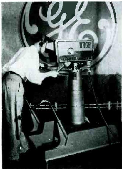
is mounted on a mobile dolly and may be operated with fingertip control. Acceptable pictures can be obtained at 50 foot-candles and f/3.5.
