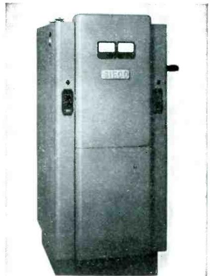
continuous output of 15 kw and features pushbutton operation. No tuning or other manual adjustments are required. Frequency of operation is 27 mc.
