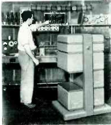
THE HARVEY-WELLS Decade Units are created to save time and expense in the laboratory, school or workshop on DC or low frequency AC electrical circuits, and are new and unique in both design and application. They use the Cannon Electric Laboratory and Switchboard fittings shown below.
