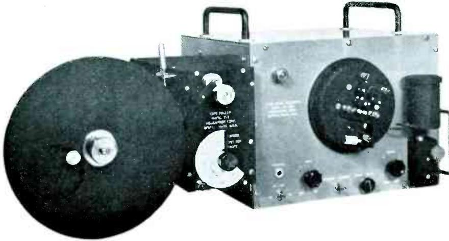
The model MA-126 series recorder represents a complete, self-contained high speed ink tape recording system. The Mecanitron recording head represents a new departure in moving coil design. A lightweight, rugged coil of eight ohms impedance is driven by a special polar, pulse amplifier.
