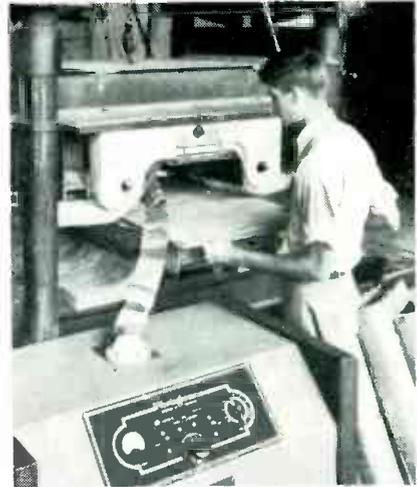
Two plys of birch or poplar and one of mahogany are glued together to form the cabinet front. A 5-kw, 5-mc Westinghouse generator is used
