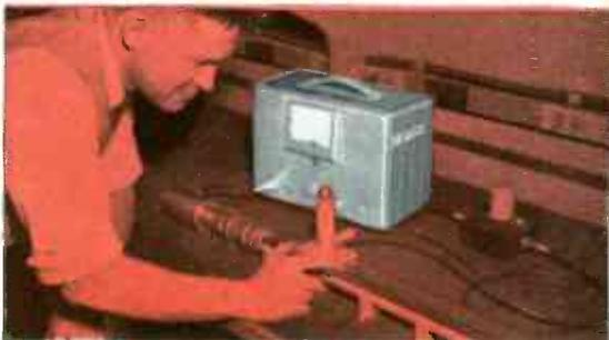
THE RCA WV-73A AUDIO VOLTMETER is a sensitive high-impedance VTVM capable of readings from 0.001 to 1000 ac volts over a range of 20 to 20,000 cycles. Logarithmic scale and overlapping attenuator assure accuracy even when pointer is at either end of scale.
