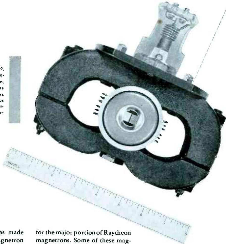
● Micro-wave radar was made practical by operating magnetron tubes in the constant field of permanent magnets. For only with this unchanging magnetic field could frequency stability be obtained. Thus a whole new frequency spectrum was opened up—and a vast new electronic market developed.
