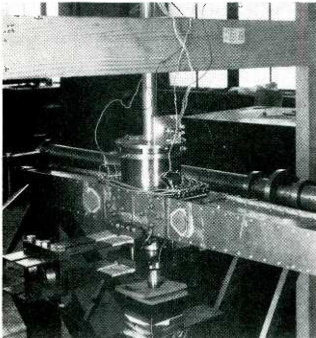
Acceleration tube, base of which can be seen projecting from its support, and gages attached to sides of simulated wing record vibrations produced by landing impact
