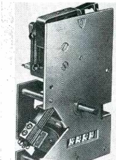
centrally wired music station. The unit features a Series 15 magnet, standard counter, wire-arm counter actuating assembly, with a midjet contact assembly having single-pole double-throw and single-pole single-throw switch combinations.
