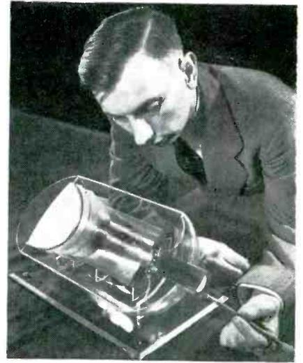
Cutaway view of the image amplifier tube. Its principle of operation is reminiscent of the Sniperscope and Sniperscope used for infrared viewing during the war
