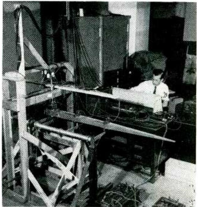
Effects of impact produced in model plane when its landing pin strikes rubber pads representing the airfield are being measured by Walter Ramberg at the National Bureau of Standards
