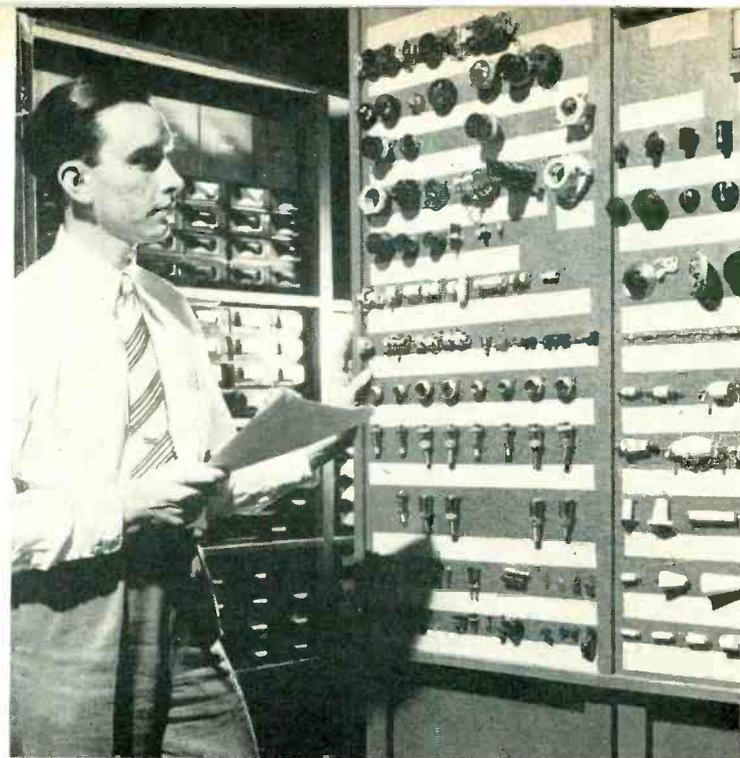
**HELP-YOURSELF STOCKROOM**—For engineers who like to pick and choose, this Transmitter lab stockroom ranks tops in popularity. Cabinets have numbered drawers, and samples of parts are mounted on boards having corresponding drawer numbers
