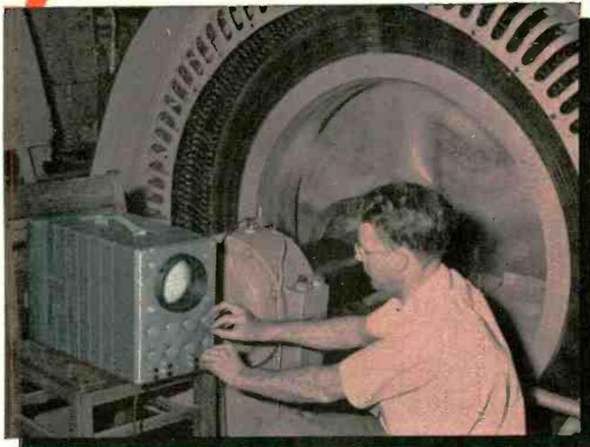
**Heavy-duty, general purpose (WO-60C)**—A “work horse” that withstands shock, dampness, dirt, fluctuating voltages. Plug-in (5") C-R tube permits change to various screen persistencies. Vertical and horizontal amplifiers practically identical. *Useful range:* 0.5 to 300,000 cycles. *Frequency response:*  $\pm 10\%$  from 5 to 80,000 cycles. *Sensitivity:* 0.056 peak-to-peak volt per inch. Exceptionally good phase-shift characteristics. Shown above measuring the vibration of a synchronous motor.
