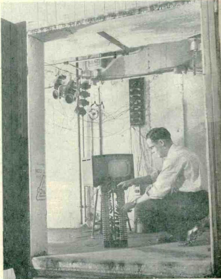
**HOT BOX**—Here receivers and components can be tested or operated for hours at temperatures up to 150 F and humidities up to 100 percent, to simulate ambient conditions encountered in any part of world where electronic equipment is used
