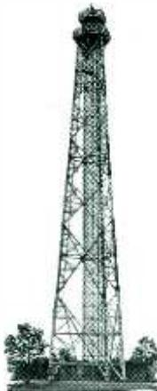
Built for microwave research . . . capable of withstanding wind velocity of 100 miles per hour . . . suitable for many uses. Triangular base 40 feet per side. Includes 180 feet of Cyclone fence, tubular steel elevator tower, 3 hp. elevator motor, approved lightning rod system . . . enclosed room at top. Readily demountable for shipment. Address inquiries to Radio Sales Department
