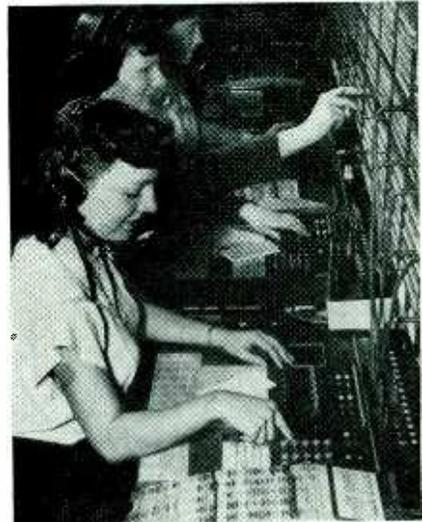
Ten keys on each of these switchboards in New York City permit the operator to ring telephones in many cities without the aid of other operators
