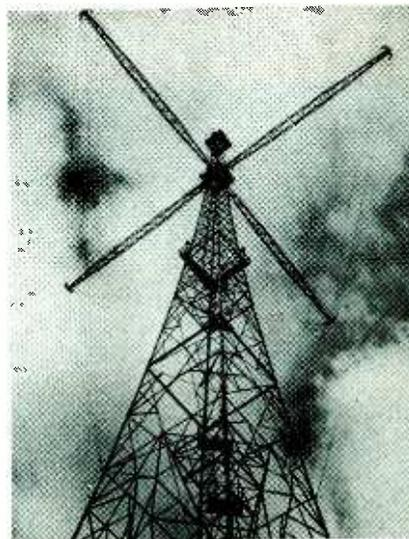
A view of the 325-ft steel lattice transmitting tower at the master station of the Lane Identification system, Puckeridge, Herts., England. Transmissions go out automatically at one-minute intervals 24 hours a day, seven days a week, so ocean-going ships approaching Britain can fix their position and set their receivers for the subsequent voyage up channel
