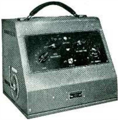
**An Electronic Replacement For Sensitive Galvanometer Systems**
