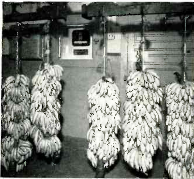
FOOD INDUSTRY Banana-ripening temperature is regulated by electronic controller on back wall, using vacuum-tube action to position steam valves accurately. This type of device indicates but does not record
