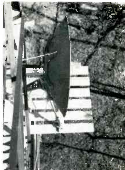
View of 2,000-mc four-foot reflector mounted on a scaffold below the cabin of the fire tower
