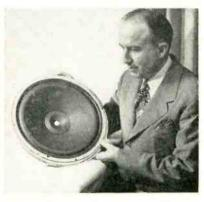
drives the small cone section to produce the high frequencies; and a 2-inch voice coil drives the large cone section to produce the lower frequencies. The unit employs a 2-pound Alnico V magnet.
