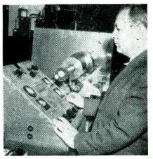
L. L. Marton of NBS at control panel horizontal experimental electron microscope used with his electronoptical shadow method of exploring and measuring small-dimension magnetic fields. Image appears on circular fluorescent screen above and to right of control panel
