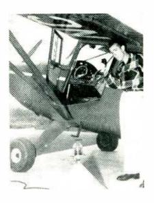
By switching the carrier of his transmitter on and off seven times in rapid succession, the pilot turns on the airport's landing lights as he approaches the field
