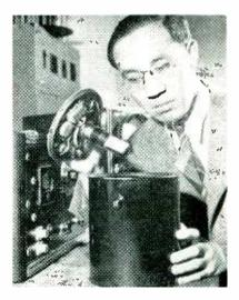
Tiny atom-smashing neutron counter being inspected by Kuan-Han Sun, who developed it jointly with W. E. Shoupp of Westinghouse Research Laboratories
