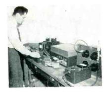
Set-up at National Bureau of Standards for noise figure calibration. At left arm of tee is the noise diode, and the right arm is a two-terminal network simulating the source. At right is a precision attenuator with a voltmeter directly in front of it
