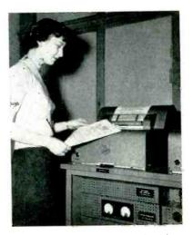
FIG. 2—Transmitted copy feeding from the recorder at a speed of <sup>1</sup>/<sub>4</sub> inch per second
