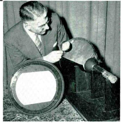
Cutaway view of tricolor tube from rear, showing aperture mask. Holes in mask, 200,000 of them each 9 mils in diameter, are formed by photoengraving process
