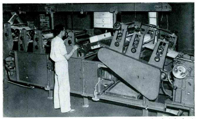
A commercial metal detector used for inspection of chewing gum. Inspecting coil is shown mounted on the machine in about the center of the picture with control box directly above it
