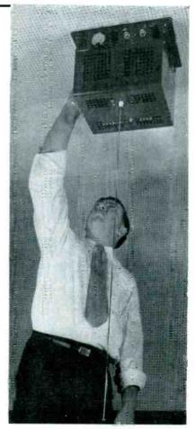
Transmitter is hung from ceiling as near center of studio as possible. Forty-inch whip is electrically short for 27 mc but inefficiency can be tolerated because of reserve of power available
