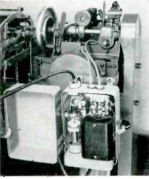
**SLOW, CUSHIONED AUTOMATIC START** Electronic speed-control automatically and smoothly accelerates the winding arbor to required speed and maintains it. No "jockeying" needed by operator. Wire breakage is minimized, tension is uniform.
