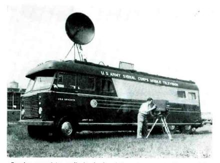
Complete transmitting studio for the Signal Corps is equipped with a specially constructed operating desk for the portable monitoring, control and power supply units used with the field ty cameras
