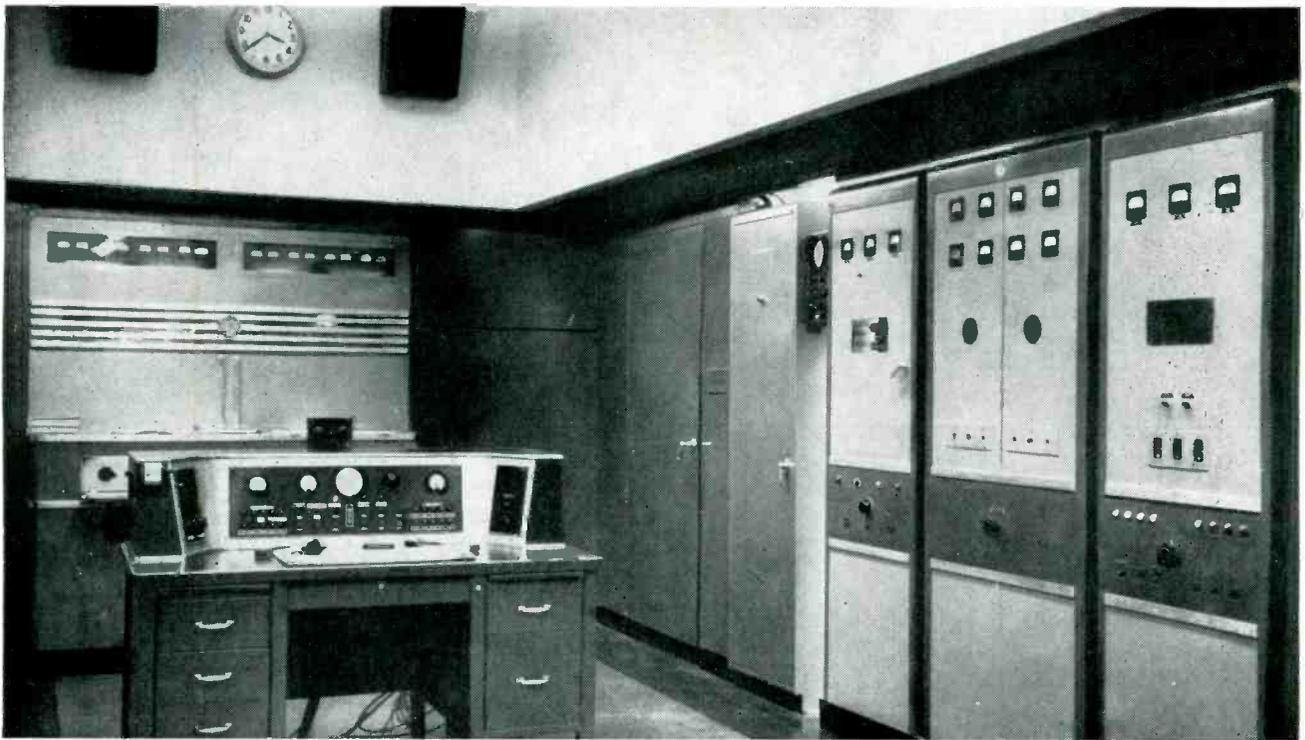
Complete emergency television transmitter with filaments lighted. In event of main transmitter failure, operator flicks toggle switch and moves chair to emergency console. Coaxial cable run starts behind false wall back of clock and continues around to right. Tall cabinet to left of oscilloscope houses 2,000-mc link that programs Bridgeport uhf experimental transmitter
