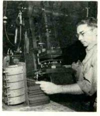
Punching of steel angle braces for 20inch picture tube supports is speeded up by use of a Verson Sheet Floater to keep the top sheet of the unpunched stack at least one finger-thickness above the others, at the CBS-Columbia plant in Brooklyn. Five horseshoe permanent magnets behind a smooth steel plate do the trick
