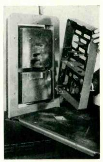
Fixture and stencils for placing lettering on both sides of a complicated chassis in one spraying operation. Stencil for bottom of chassis, in upright part of fixture, has cavities for under-chassis projections. Stencil for top of chassis, on hinged frame resting on table, is brought up after chassis is inserted in fixture
