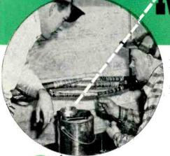
Veteran splicers in the Underground Department like Natvar splicing kits, because they provide exactly the right number of rolls of v.c. tape cut to proper lengths and widths, and exact quantities of other materials required for the job. Engineers and foremen like the kits because they give close "quality control" of the splicing operation, with a minimum of waste and spoilage.
