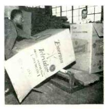
Roller on simple wood frame facilitates tipping over consoles in cartons at Emerson plant
