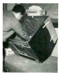
Padded bench at CBS-Columbia. Safetyglass plate being installed here was first cleaned with special lintless industrial absorbent tissues
