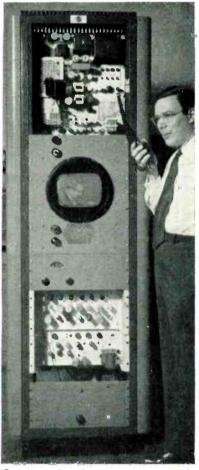
Activities of roving cameraman are directed over radio link from this control station, which picks up the video and audio program signals broadcast from the pack set
