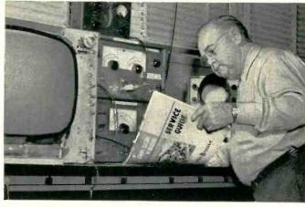
LABORATORY TIME-SAVER. Accurate, hand-calibrated dial permits development engineer to do 95% of his work without frequent reference to the crystal calibrator. No listening for or counting of "birdies." No time wasted making allowance for a printed dial, since the hand calibration matches precisely its associated capacitor.
