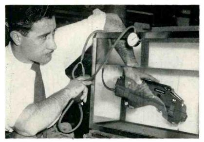
New method of testing for leaks in housing of military radio unit
