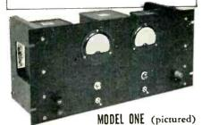
is a 300 vdc, 0-300 ma supply, conservatively built for years of reliability, and featuring a specially stabilized high-performance electronic regulator.
