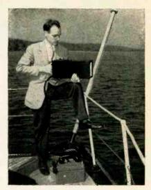
Radar identification system shows harbor control radar which ship is which. Pulses picked up by microwave horn (center) are fed back through communications radio set
