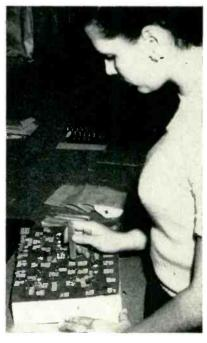
Use of fishpaper template to speed positioning of rubber stamps for marking a chassis
