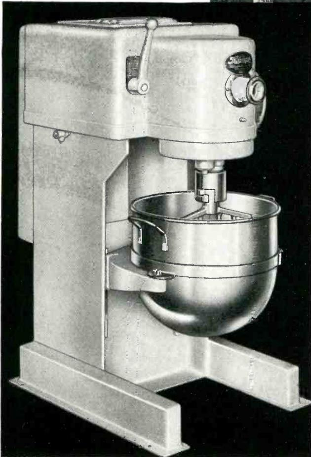
This Triumph vertical “kitchen” machine is used by the Navy for everything from mixing dough to cutting French-fried potatoes, grinding coffee, sharpening cutlery.
