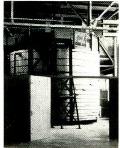
White-cedar sonar test tank at NADC is used in calibration of barium-titanate transducers
