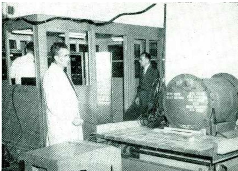
Instrument container with accelerometers attached mounted for acceleration-table test. Table connects to vibration recorder housed in shelter, left
