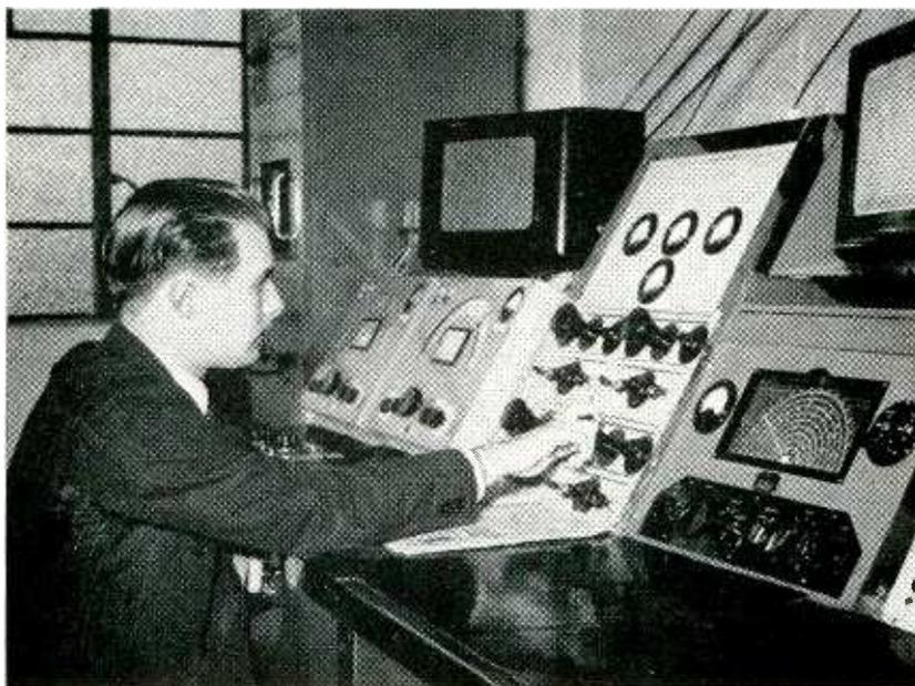
Television sound signals at audio frequency are passed to this control room for monitoring and redistribution over the feeders
