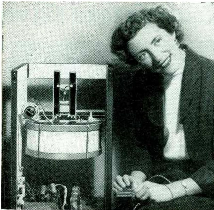
Operator playing the electronic drum. The electromagnetic system is mounted above the drum diaphragm
