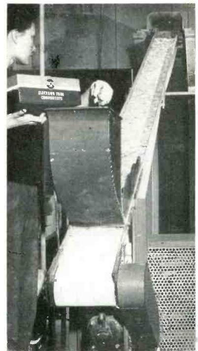
Loading mica spacers into hopper that distributes them over conveyor belt of sorting machine
