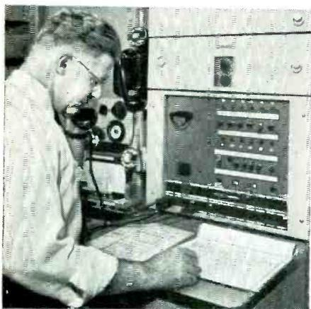
Alarm-receiving bay in town. Lights on a chart report on 42 separate conditions affecting service. Telephone is to communicate with maintenance crews. Eleven alarm centers across the country cover all 107 radio-relay stations. Stations too far off the beaten trail for wire connections signal by very high frequency radio.
