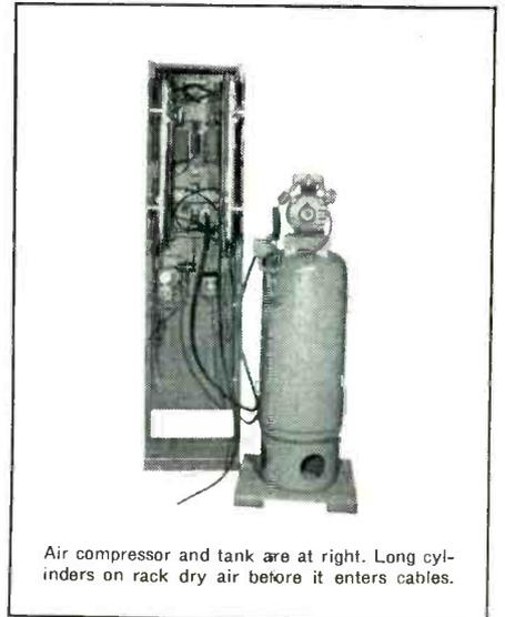
Air compressor and tank are at right. Long cylinders on rack dry air before it enters cables.
