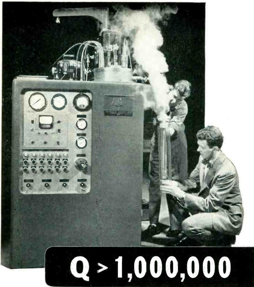
Resonant circuits with Q's in the range of millions are one of the many practical applications of low-temperature techniques and phenomena being studied by laboratories equipped with our Collins Helium Cryostat. With this reliable equipment for the production of liquid helium, phenomena known to occur in the neighborhood of Absolute Zero are now being exploited for useful purposes.
