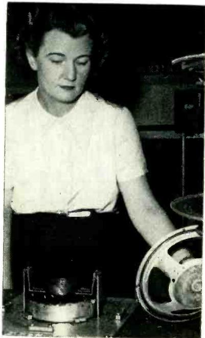
Operator demonstrates use of fixture for applying ring of red thermosetting cement to speaker frame for anchoring spider. When she releases lever in right hand, the ring and its strap iron side supports will drop down into the pot to pick up cement for the next speaker
