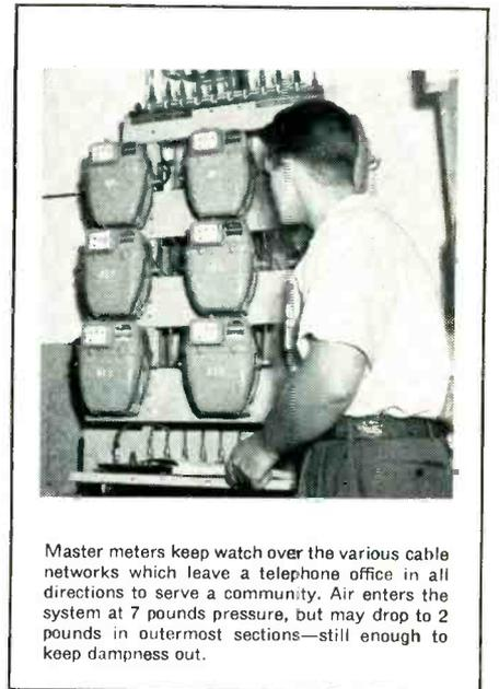
Master meters keep watch over the various cable networks which leave a telephone office in all directions to serve a community. Air enters the system at 7 pounds pressure, but may drop to 2 pounds in outermost sections—still enough to keep dampness out.
