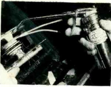
Applying household cement to television transformer with oiler
