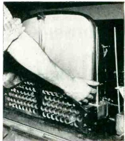
Adjusting position of picture tube with respect to fixture locked in position over front of television receiver chassis. Drilled holes lighten weight of fixture without impairing the rigidity
