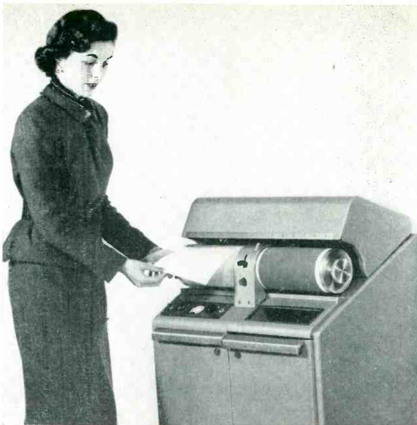
Placing copy of printed form on cylinder of Stenafax machine. Finished stencil, ready for use, is obtained in 6 minutes on right-hand cylinder
