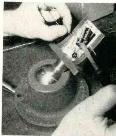
Combination slide and peg fixture for terminal board subassembly work in connection with subminiature equipment. Terminal board slides in grooves, going down between metal spacing rods inserted in bottom of fixture. Rods on one side serve to space silver-button mica capacitors off the chassis, and rods on the other side space four parallel ceramic capacitors off the chassis
