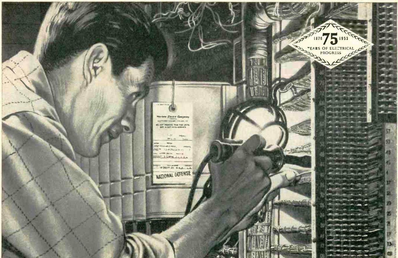
Western Electric installer in an aircraft plant connecting telephone equipment with a G-E soldering iron.
