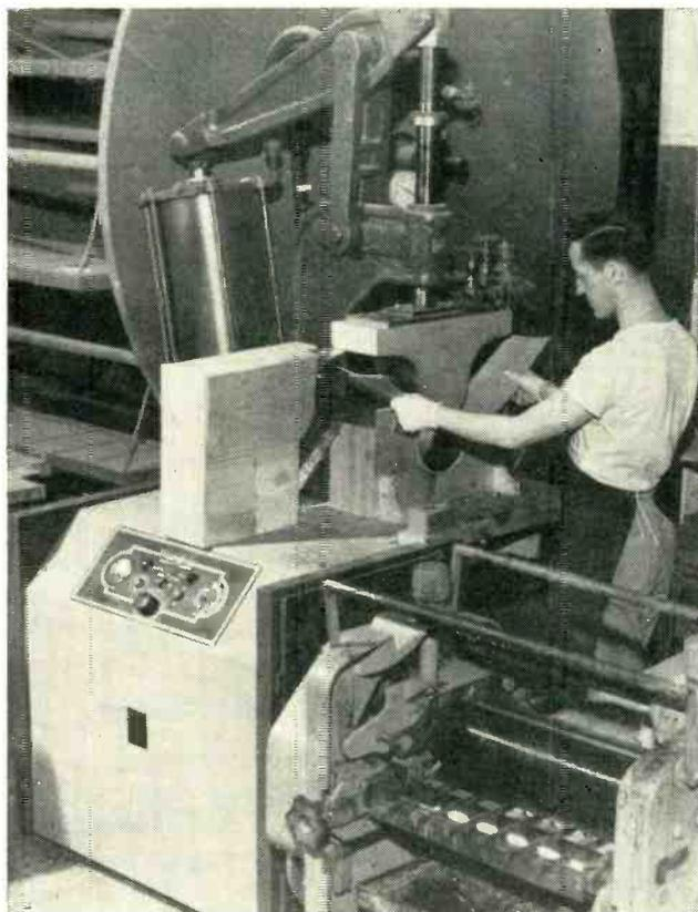
**CURVES**—Forming and glue-curing laminated cases for clocks with Westinghouse equipment. Glue is automatically applied to individual laminations by roller of machine in foreground
