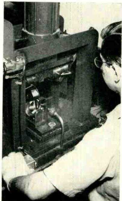
Pressing 90-degree yoke coils to shape
