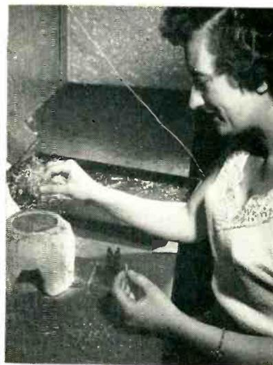
Pigtail is dipped through solder pot with a sweeping motion to minimize pickup of dross on surface. Body of capacitor is in left hand, ready for quick application to lead
