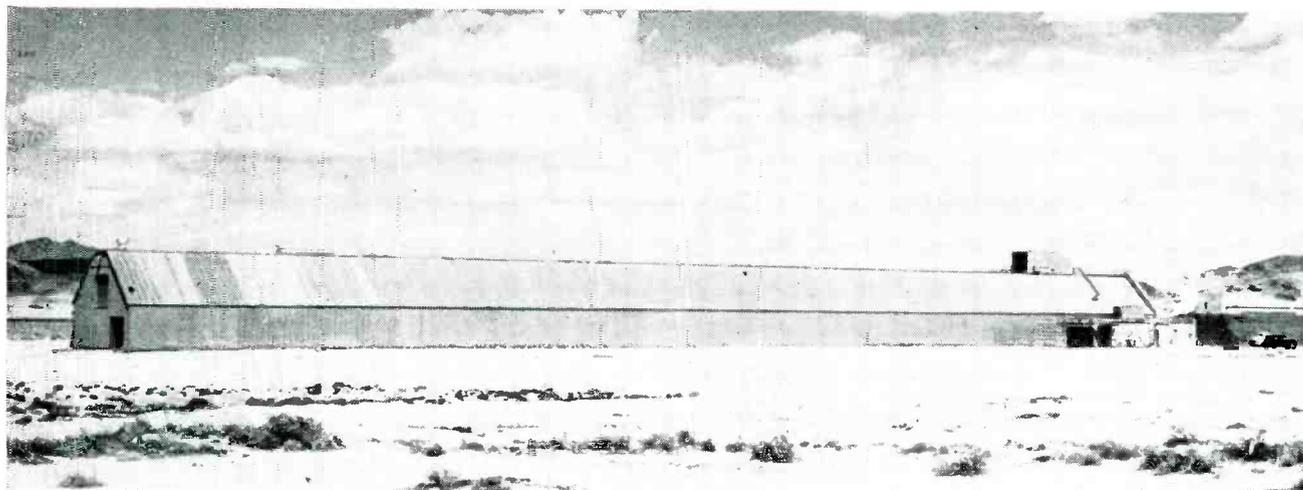
NOTS Aeroballistics Laboratory at Inyokern. Gun platform for firing rockets is at right end along with control room; missile stop is at left end of building
