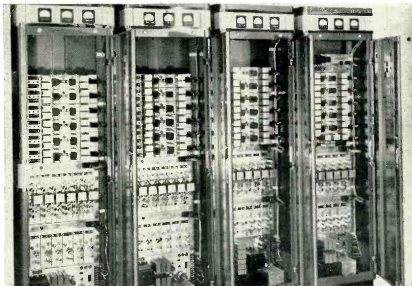
Complete 24-channel system. From top to bottom, each cabinet contains: six voice-channel terminal equipments, six subcarrier receivers and transmitters, and power supply
