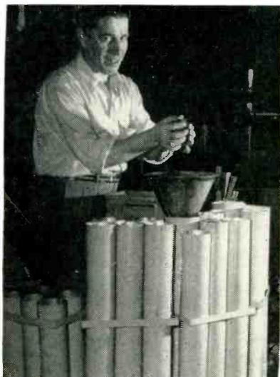
Loading hoppers of rotary riveter
