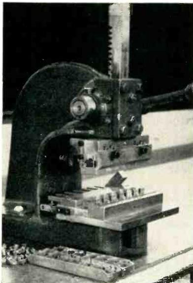
Arbor press modification for inserting subminiature sockets in chassis, as used at Utility Electronics
