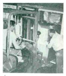
Using fork truck to move plasticwrapped section of radar unit into reusable steel shipping container, especially designed to receive one complete fire-control unit
