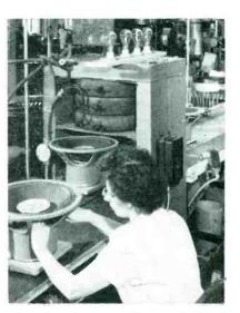
Assembly line for high-fidelity loudspeakers, with 2<sup>1</sup>/<sub>2</sub> ton magnetizer straddling conveyor belt that runs over top of bench. Light beam goes diagonally through magnetizer from right front of bench to phototube at left rear. Surgeabsorbing lamps are on top of magnetizer frame.
