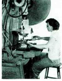
Typical installation of two-hand clutch control on Niagara punch press used in producing electronic components
