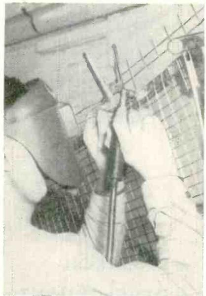
Top and bottom edges are welded on face of screen. Excess screening is clipped one inch beyond tubing, rolled over and tacked along reverse side
