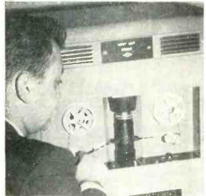
Microfilmed documents previously marked are read off by flying-spot scanner in new technique developed for computer input
