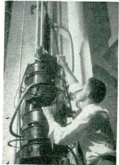
Tests show that the klystron has a power gain of 38 db. Plate efficiency of 43 percent has been measured with as high as four megawatts of peak power output. Research carried on from 1948 to 1950 has recently been declassified.
