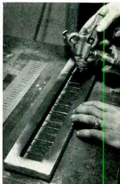
Spraying resistor board with DeVilbiss spray gun, using stencil frame having wires that automatically press stencil against board
