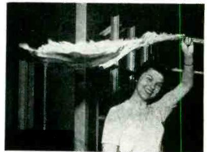
Scarf held in open door illustrates how air pressure keeps dust out of radar tube assembly area
