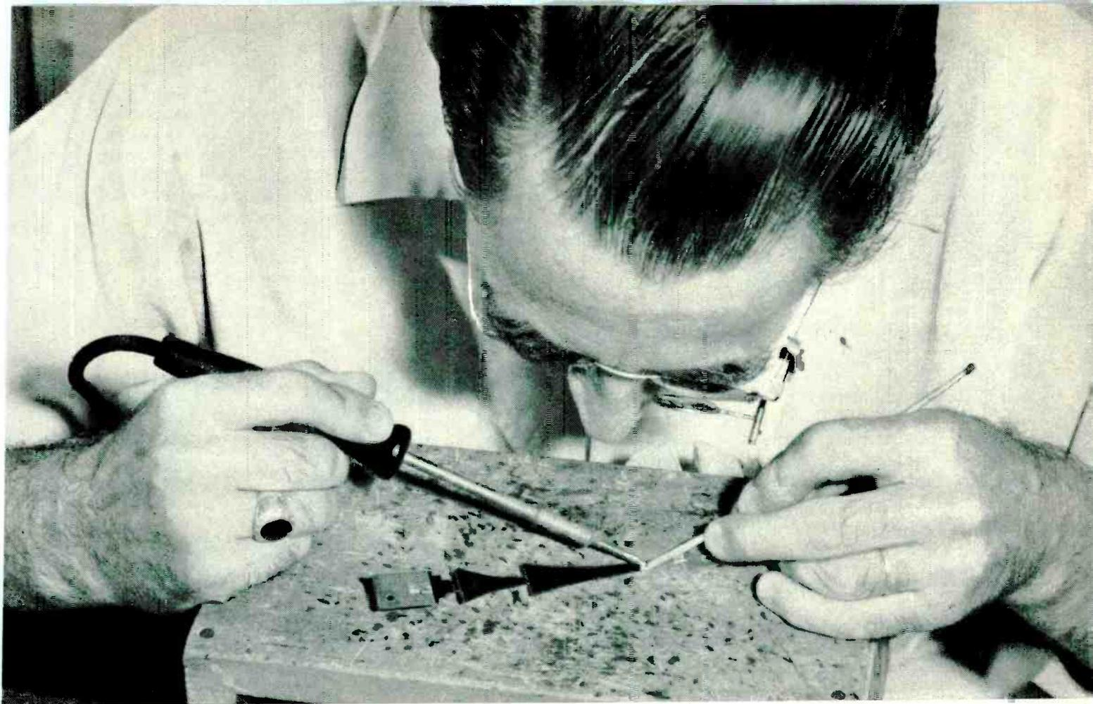
**CRAFTSMAN USES JEWELER'S GLASS** and the G-E Midget iron to solder a potentiometer joint the naked eye can't see. Equipped with a pencil-fine tip, the Midget can solder delicate
