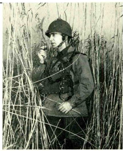
Receiver-transmitter is strapped to chest and power pack is on back, with antenna on helmet. Total weight is 26 lb. All units are waterproof, with controls accessible through watertight plugs and fittings
