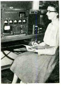
Production-bench setup for testing packaged servo amplifiers
