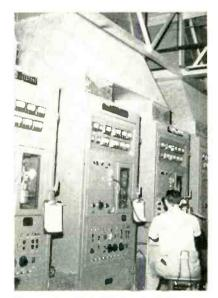
Four of the 64 hydrogen thyratron test sets from which hot exhaust air is ducted into building's heating system
