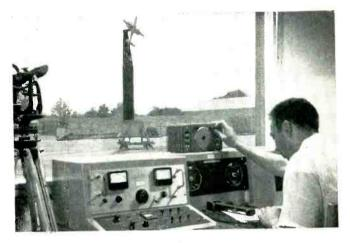
Electronics Research Engineer Irving Alne records radiation antenna patterns. Twenty-two foot plastic tower in background eliminates ground reflections, approximates free space. Tower is of Lockheed design, as are pattern integrator, high gain amplifier, square root amplifier, logarithmic amplifier.
