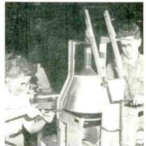
Bolting mounting yoke in position on color picture tube
