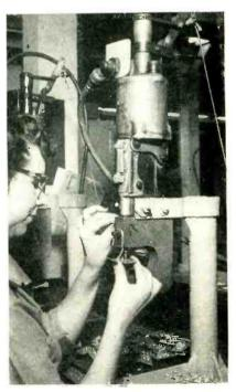
Manual method of staking turret terminals in plastic boards, using air-actuated squeeze-type riveter
