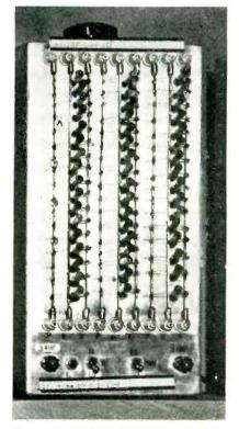
Burn-in rack for 50 miniature tubes. Temporary lap joints are used for soldering tube leads to the vertical busbars
