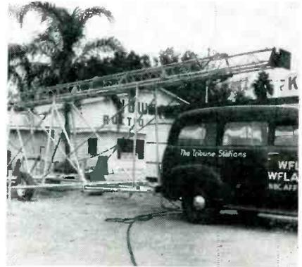
FIG. 1—Trailer carrying tower is located at desired spot. Outriggers keep unit steady while tower is raised in about three minutes
