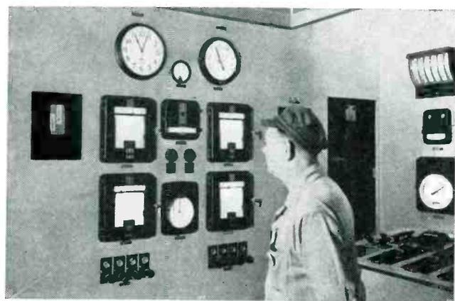
Indicating panel of power station has linear and circular self-balancing recorders to record steam-gas and air, feedwater and other temperatures on continuous basis
