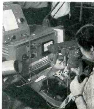
Automatic welding setup used for welding tap on precisely the correct turn of a precision potentiometer
