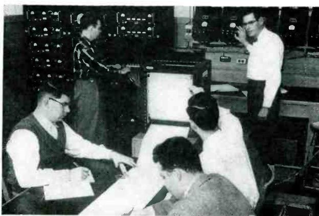
Data recorded on multitrack paper-tape oscillograph, at receiving end of telemetering link, is read off by engineering staff for subsequent interpretation and evaluation
