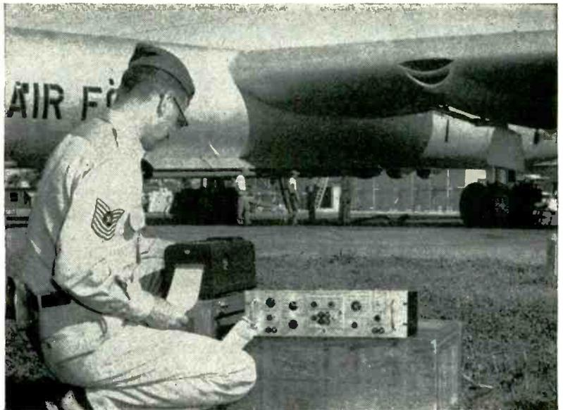
**Checks bomber refueling.** Brush instruments are rugged and durable, maintain accuracy in field use. Here they record surge pressures in gas tanks of a Strategic Air Command B-36 during refueling. For top performance, bomber must be refueled in a hurry, yet flow rate of 600 gallons per minute posed a pressure problem. Brush Recording Systems provided necessary facts.
