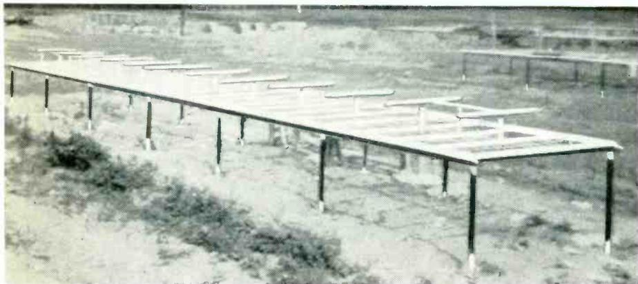
Satellite tracking antenna is mounted on jack-type posts to permit leveling
