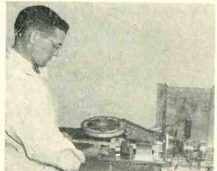
Prototype system developed by Stanford Research Institute duplicates from original text at the rate of 17,000 characters of elite type a second. Signals received on a cathode-ray tube charge a paper ribbon. When dusted with black powder, a sufficient amount clings to the charged areas. The powder is then heated and pressed into the paper to give a permanent record
