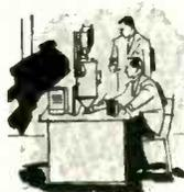
◀ Timing photo-cell controlled exposures in automatic photo printing machine at Eastman Kodak Co.
