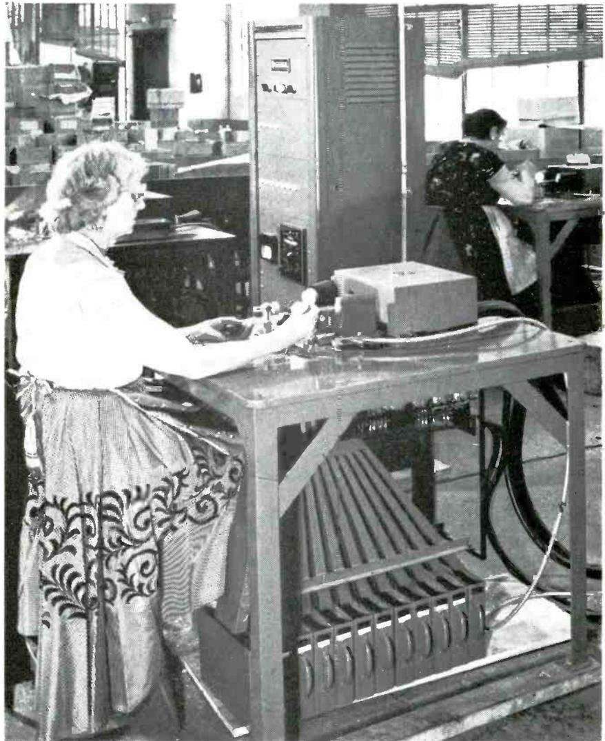
At sorting position, operator now merely inserts mica sheets one by one between gaging contacts. Electronic gage measures thickness to thousandth of inch and drops sheet into proper receptacle below. Control equipment is in relay rack at rear
