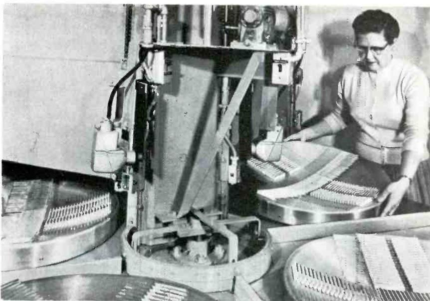
Loading tray of subminiature guided-missile and radar tubes on turntable of new automatic x-ray machine. X-ray tube is in heavy metal shield box at rear over turntable
