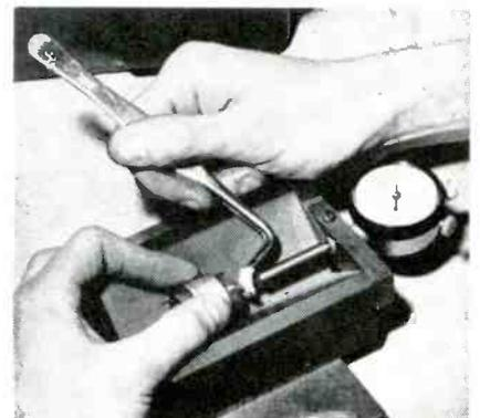
Method of using fixture for checking end play of precision servo motor
