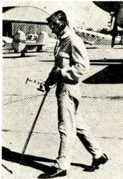
Operator traces underground cable at airport installation and pin-points cable fault. The detecting-element coil is mounted on the telescoping boom connected to the amplifier-indicator case. Signal strength is indicated on an output meter and headset monitors the output
