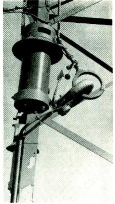
Tower insulator, showing how one electrode of original ball-gap was replaced with point and gap reduced to  $\frac{1}{8}$ th inch for minimizing effects of lightning
