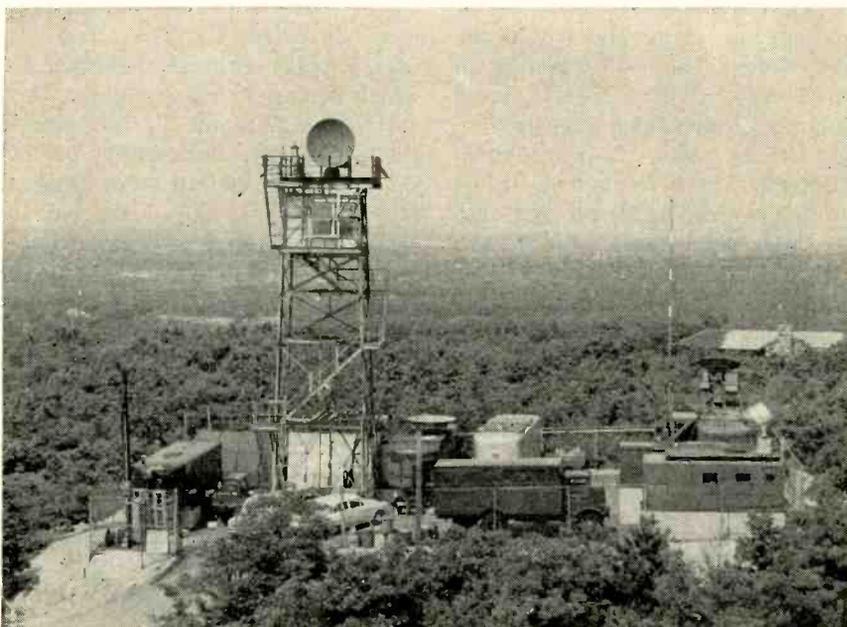
**FRONT COVER**—Radar weather station at Milton, Mass. has four radars operating from 0.86 to 3.2 cm. has observed many of the angel echo phenomena
