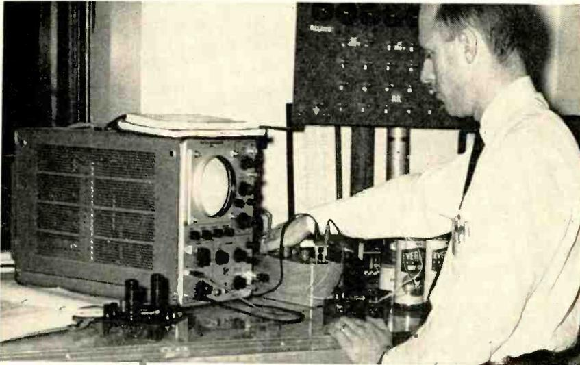
Waveforms of magnetic inverter are checked on oscilloscope and effects of bias variations determined
