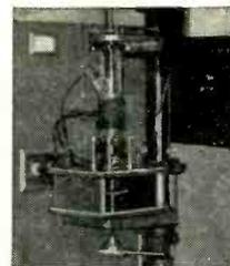
General arrangement for pulling single crystals. Induction heating coil is shown surrounding quartz tube containing crucible with molten germanium in suitable atmosphere.
