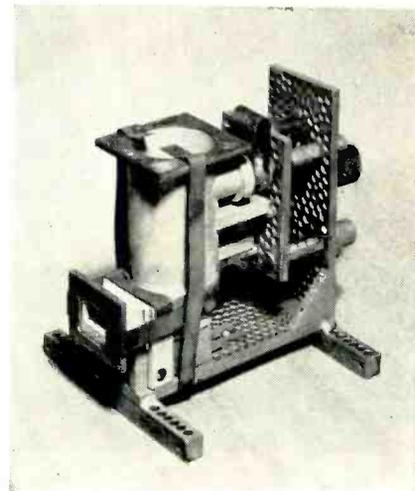
Spring-loaded fixture holds mount together during brazing
