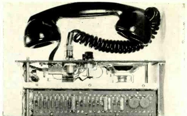
Service channel portion of level panel with telephone handset indicates simplified modular construction
