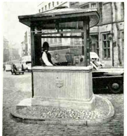
Bobby controls traffic lights by watching monitor as closed-circuit tv cameras see vehicles around bends and over bridges in Durham, England
