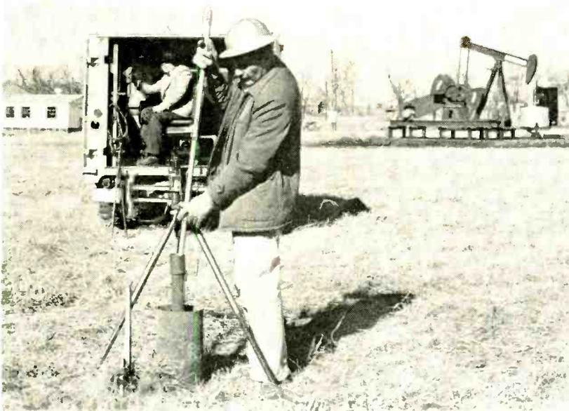
Field engineer lowers assembled gamma-ray probe into wellbore prior to beginning logging operation. In rear is mobile unit containing recording instruments
