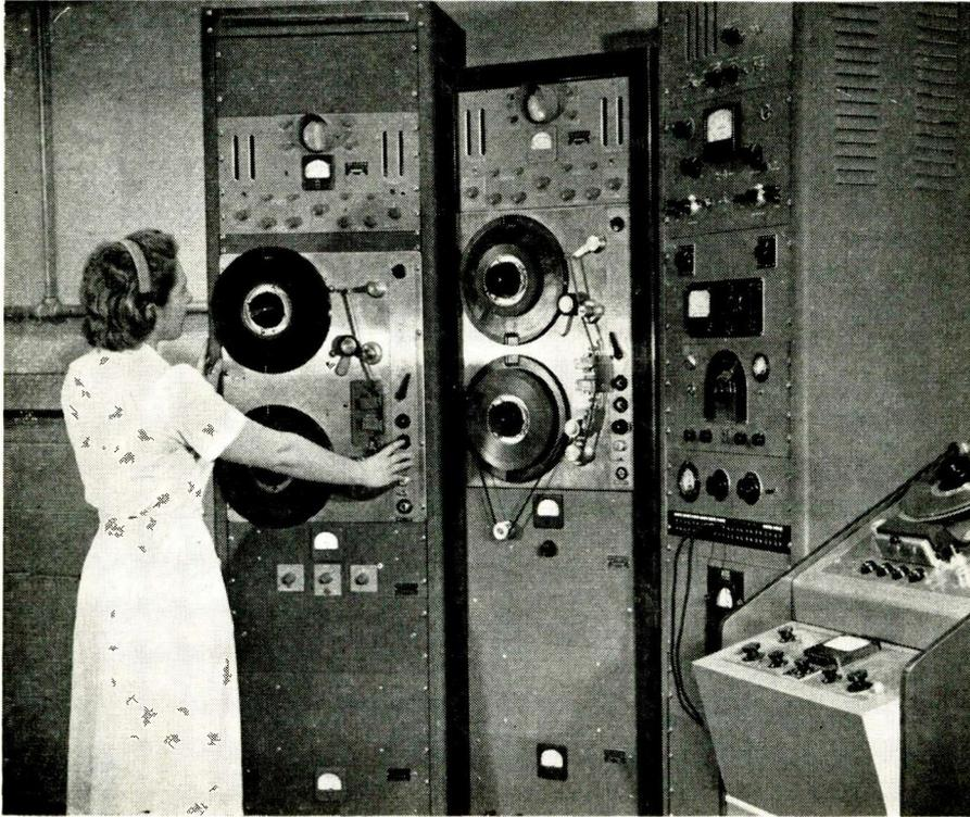
The machine above is a unique testing instrument, designed by Audio Devices engineers and installed at the Audiotape plant in Glenbrook, Conn. This Automatic Defect Counter records and plays back every inch of the EP Audiotape under test.
