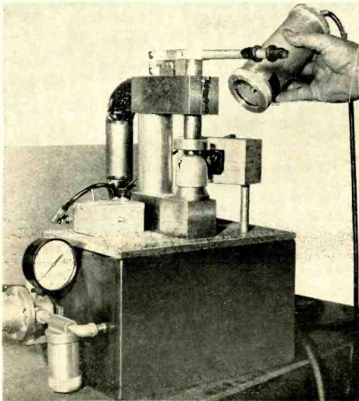
As air motor spins high-explosive charge in magnetic field, a sensitive iron probe, rigidly mounted in the plane of the barrier, picks up variations in the flux pattern and determines the concentricity of an encapsulated piece of steel which plays a key role in controlling detonation pattern of explosive
