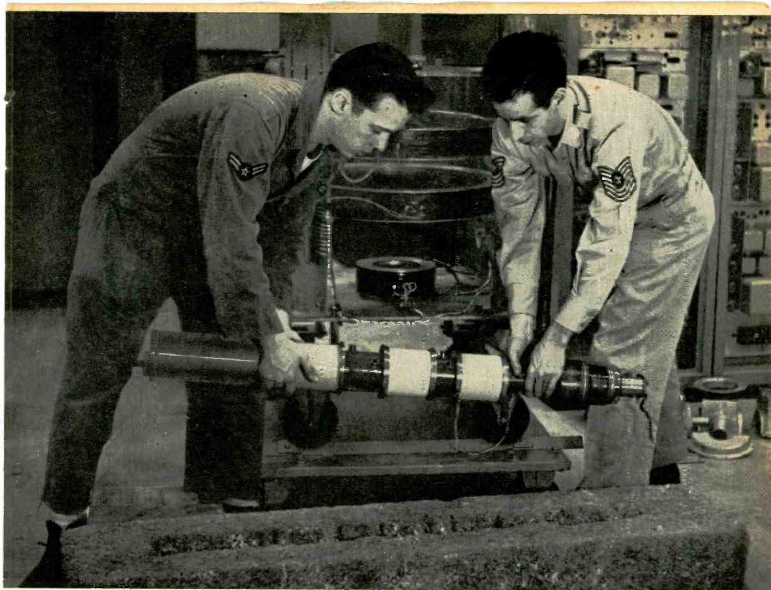
U. S. Air Force personnel remove 25,137 hour klystron from advanced Pole Vault base. Department of Defense Photograph.
