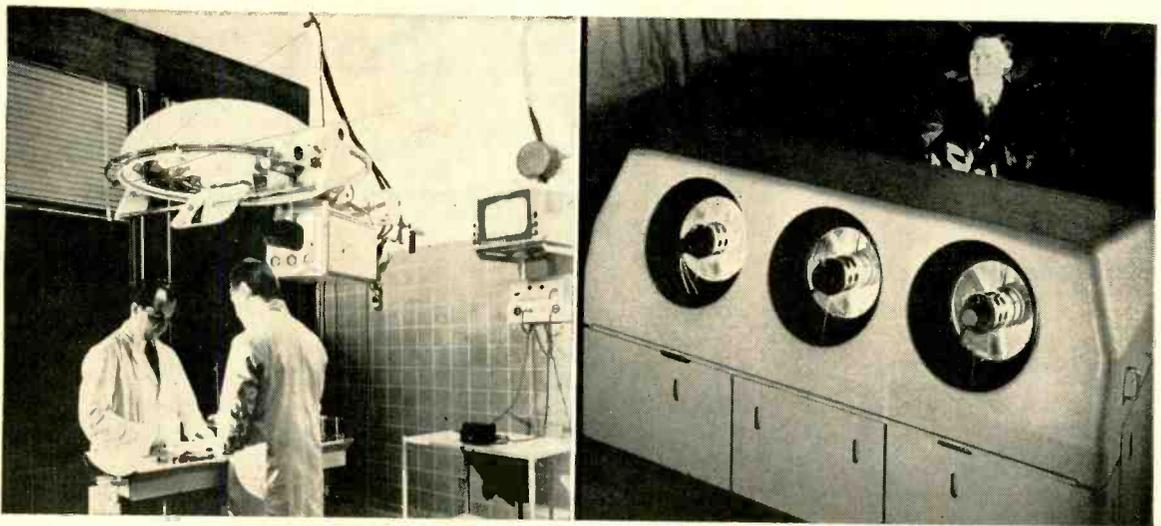
Details picked up by camera focused on filtering mirror above operating table are displayed on screen by three-barrel projector
