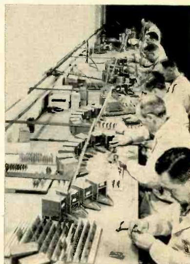
PROTOTYPE QUANTITIES of printed wiring boards are assembled at Avco's Advanced Research and Development Division, Lawrence, Mass., on small assembly lines like the one shown. In addition to purchased fixtures and feed trays, the assemblers are using 2 fixtures made in the division's shops.
