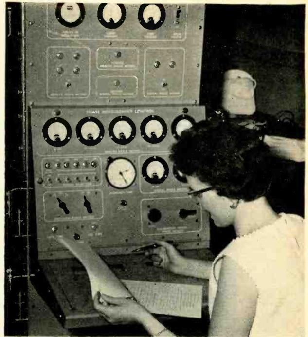
Operator, seated at console of the Minitrack data system, checks system operation
