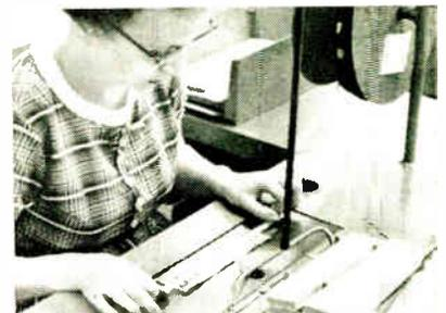
Stacking capacitor strip by hand
