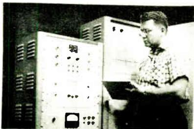
Electronic device called ASCAT (Analog Self-Checking Automatic Tester) made by Bell Aircraft tests electrical, hydraulic and pneumatic systems of missiles and aircraft. Single technician can in two minutes make same checkouts formerly requiring an hour by 10 men. Tester supplies unit being checked with predetermined sequence of d-c signals. Returned signals are compared with preset standards
