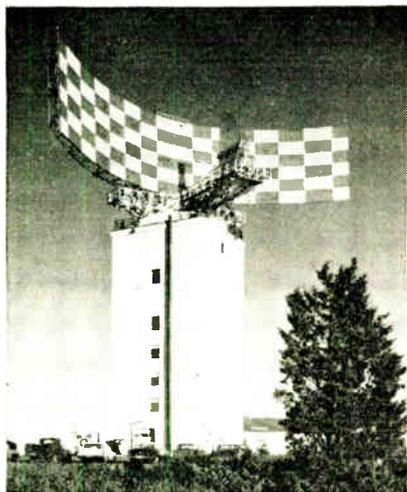
New experimental high-power search radar, designed by MIT's Lincoln Laboratory, is operating in North Andover, Mass. Radar reportedly has frequency of 400 mc with peak power of 5 megawatts. Reflector: 120 ft wide, 30 ft high
