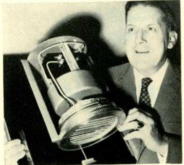
Full-scale mockup of Rocketdyne experimental ion-drive engine that will weigh about 1½ lb and produce about ¼-lb thrust. Electrical power will be supplied by nuclear reactor power generator
