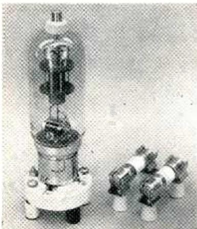
Silicon diodes and mountings require less than one-half volume of 577 diode
