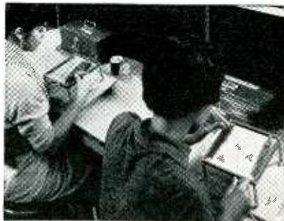
Hand wiring of memory core array. Improved methods are less tedious
