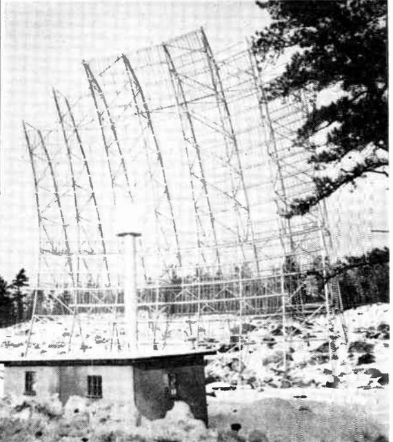
Rugged reflectors for quadruple-diversity single-sideband tropospheric scatter link are part of DEW-line extension in northeast Canada (inset). System is one of first to use parametric amplifiers in receivers
