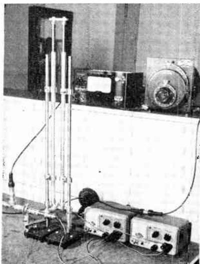
Complete bench setup for determination of maximum frequency of oscillation
