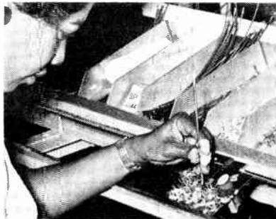
Assembler uses hollow tube tool to weave wire through slots in tube socket terminals
