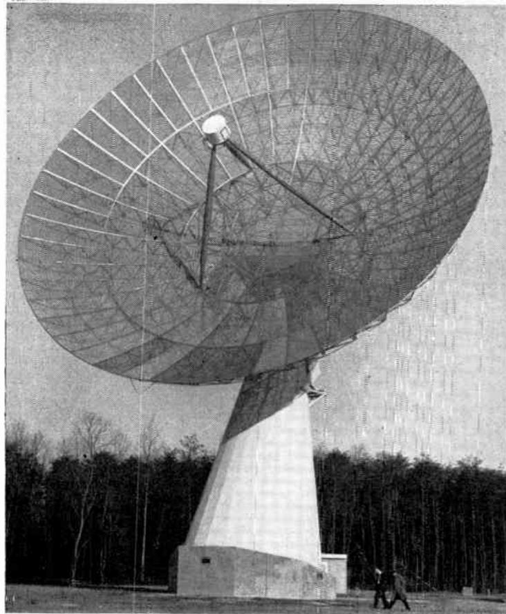
Naval Research Lab's 84-ft radio telescope at Riverside, Md., has maser at focal point
