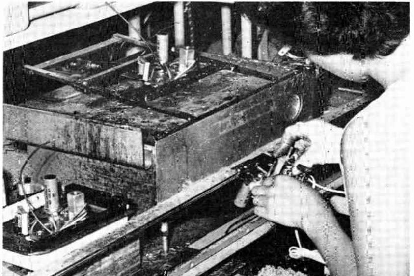
Chassis at lower left is in flux bath. The other chassis is on the cam-operated jig which lowers terminal tips and wire connections into solder bath
