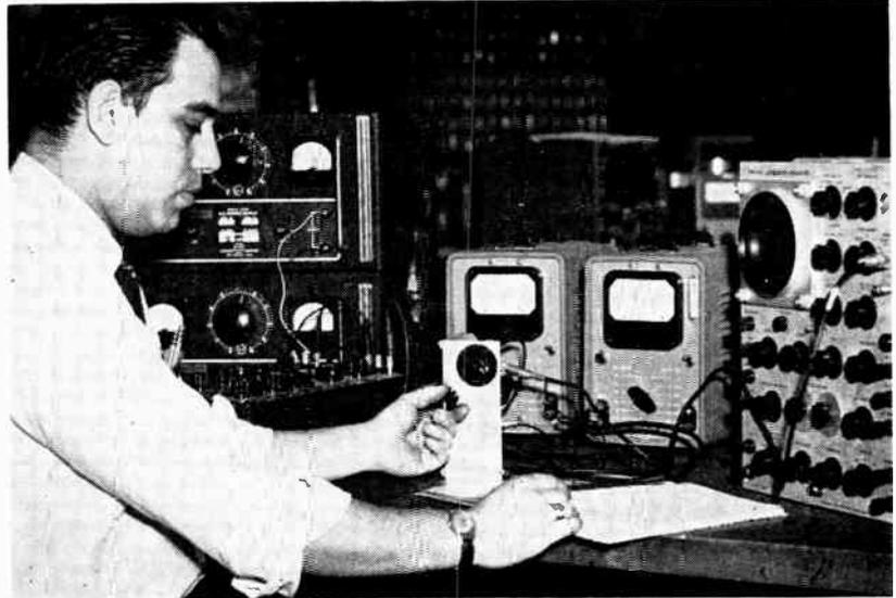
Technician obtaining test data on compensation of a loaded potentiometer
