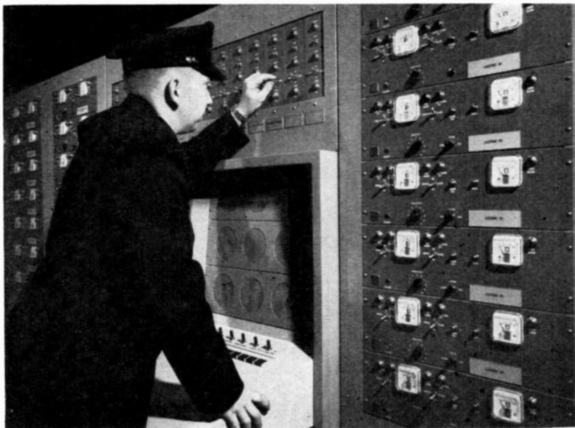
Console (center) lets guard communicate with nine points, while subsystem panels (left and right) give him security information
