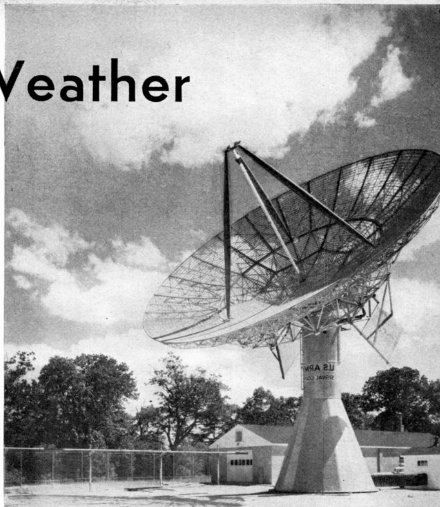
Army's 60-ft dish, being converted for automatic tracking of Tiros weather satellites, uses new lens and waveguide not shown here
