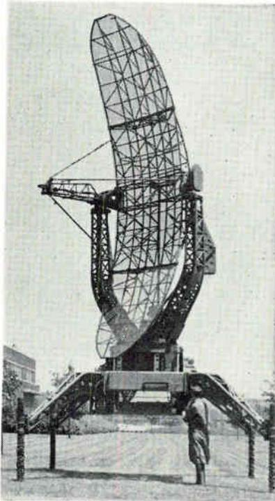
Radar set AN/MPS-16, a C-band height finder, was used in solar-noise calibration experiments.
