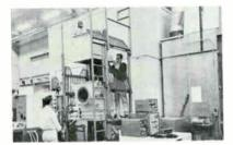
Assembling outgassing furnace around the tube
