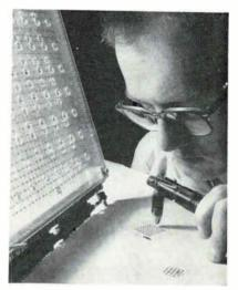
Each of 64 magnetic thin film dots on 2-inch square glass contains one piece of information. Minneapolis-Honeywell scientists have placed as many as 1,024 dots on same size glass hoping to replace ferrite core memories like that shown at left
