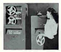
System for Signal Corps inventory control links computers in Philadelphia, Pa., and Lexington, Ky. Reel holds 25,000 transactions
