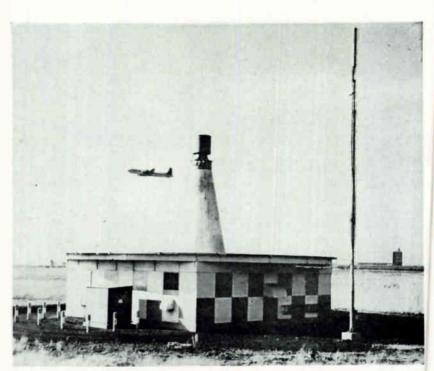
Typical station for broadcasting direction and distance information to pilots
