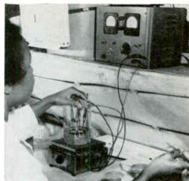
FOUR microinches of 24-karat gold coating is deposited in less than one minute in plating silicon disks
