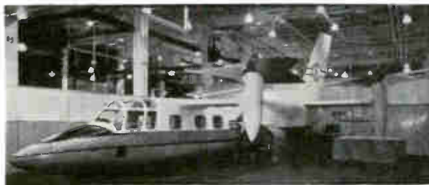
VTOL TRANSPORT uses ducted propellers in artist's illustration of research aircraft built by Bell Aerosystems Co. Speeds to 350 mph in conventional flight are expected in this military craft
