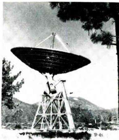
*Single 70-ton counterweight balances 85-foot telescope in any position*
