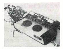
displacement metering pumps having d-c variable speed drives with rpm indicators measuring pump speeds.
