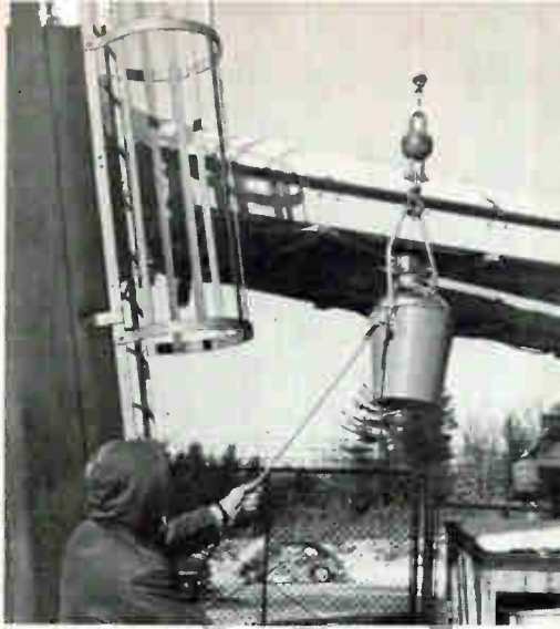
MASER dewar being hoisted to antenna
