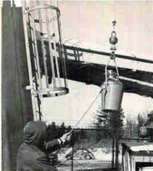
MASER dewar being hoisted to antenna
