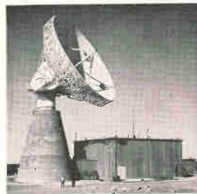
60-FOOT ANTENNA provides pencil beam for tracking reentering missiles
