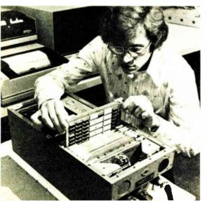
the Westinghouse computers will operate with 16-bit words at speeds of 375,000 operations per second as well as handling 32-bit, 8-bit, or single-bit increments. The DAIS processor and its read-only memory use off-the-shelf, large-scale integrated circuits. The capacity of the core memory is 64,000 16-bit words.
