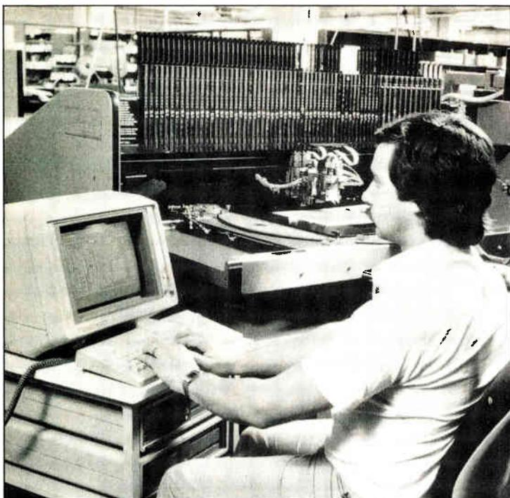
**CAD/CAM.** At Tektronix, CAD data is converted to a machine insertion program for loading a pc board with packaged ICs.
