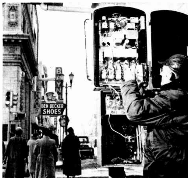
RADIO-COORDINATED traffic signal in Evansville controls downtown traffic
