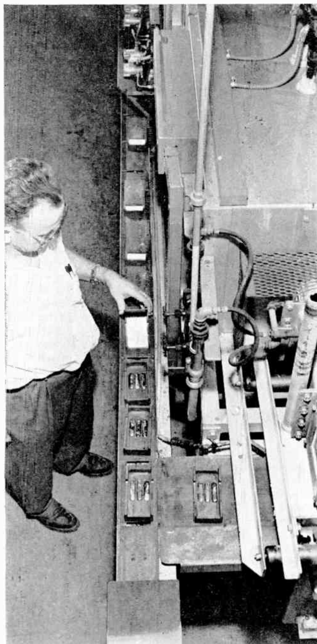
Reducing germanium in continuous furnace (GE)
