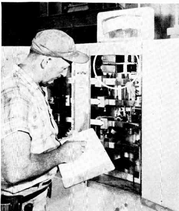
Batching scales are photocell controlled
