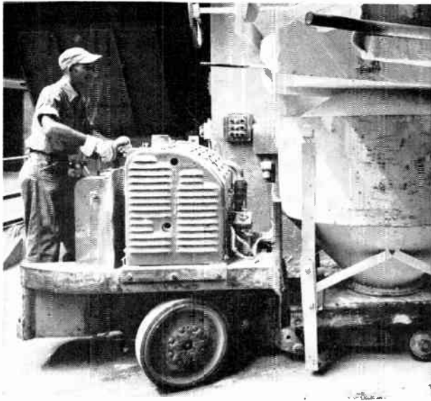
Loader (left) gets signals from batch house (right) telling how much sand and chemical to add
